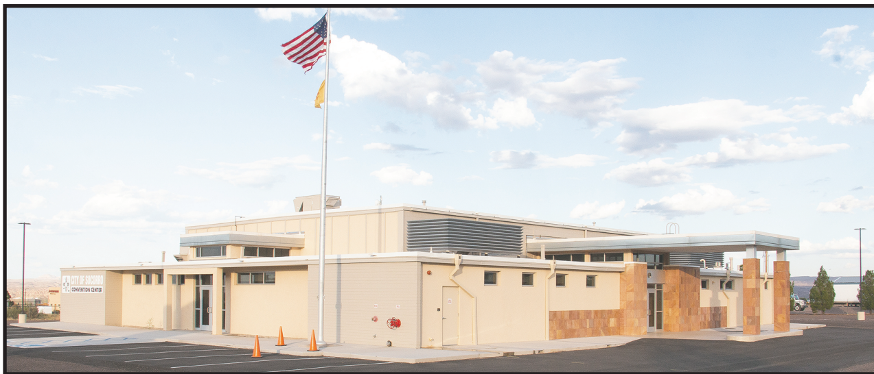
Socorro Convention Center, 1220 US Highway 60, Socorro, NM
