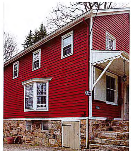
Traditional wood clapboard siding and a stone foundation define the historic character of this vernacular residence
