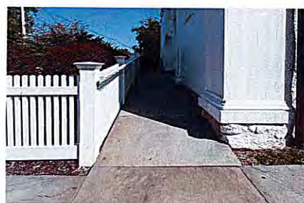
Accessible ramp added with minimal effect on historic fabric
