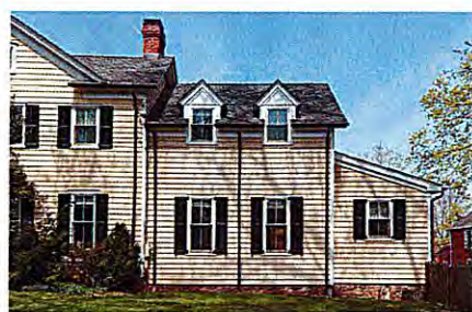
Side additions extend from the main block, maintaining original window rhythm
