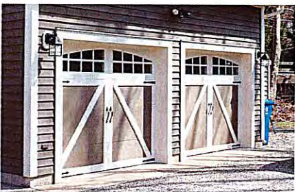
Modern overhead doors with decorative cross-bracing and divided lites
