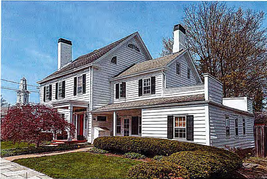
Rear and side porch enclosures expanded this Federal-era dwelling while preserving its distinctive form and decorative details
