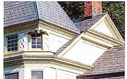
Ornate Queen Anne trim with decorative cornice brackets, dentil molding, and drop pendants
