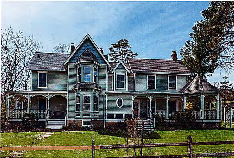
Wood clapboard siding, decorative trim, and a raised stone foundation are key components of this Queen Anne-style residence, illustrating the interplay of texture, detail, and materials
