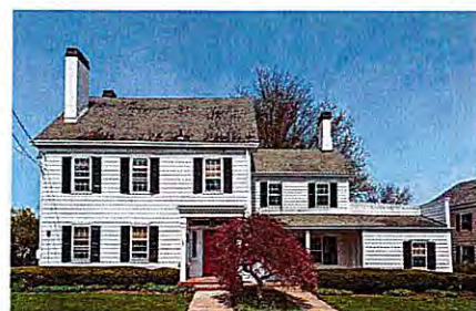
Robert M. Honeyman House | 4 Joliet St
