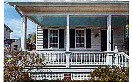
Repair and retain original materials whenever possible
