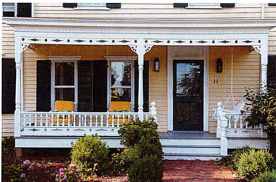
Ornamental front porch with turned posts, sawn brackets, and spindlework balustrades are important character-defining features with great influence on the character of the streetscape
