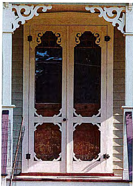
Double-leaf wood screen doors with decorative scroll-sawn panels
