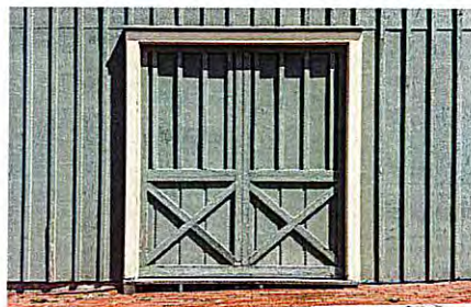
Decommissioned entry with preserved board-and-batten doors with cross-bracing
