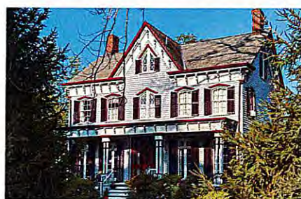
9 Old Turnpike Rd
