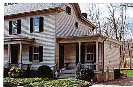
Later shed-roofed entry porch reflects early 20th-century functional updates
