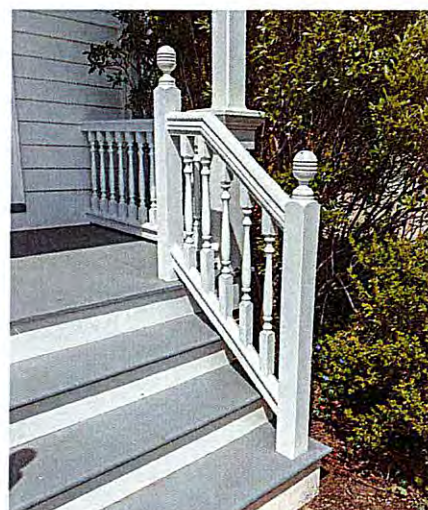
Wood stair railings with turned balusters and newel posts reinforce the historic character and craftsmanship of traditional porch entries
