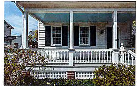
Turned balusters, square newel posts, and wood lattice skirting preserve the historic character and craftsmanship typical of 19th-century porch design
