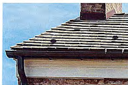
Original U-style gutters, round downspouts, and snow birds
