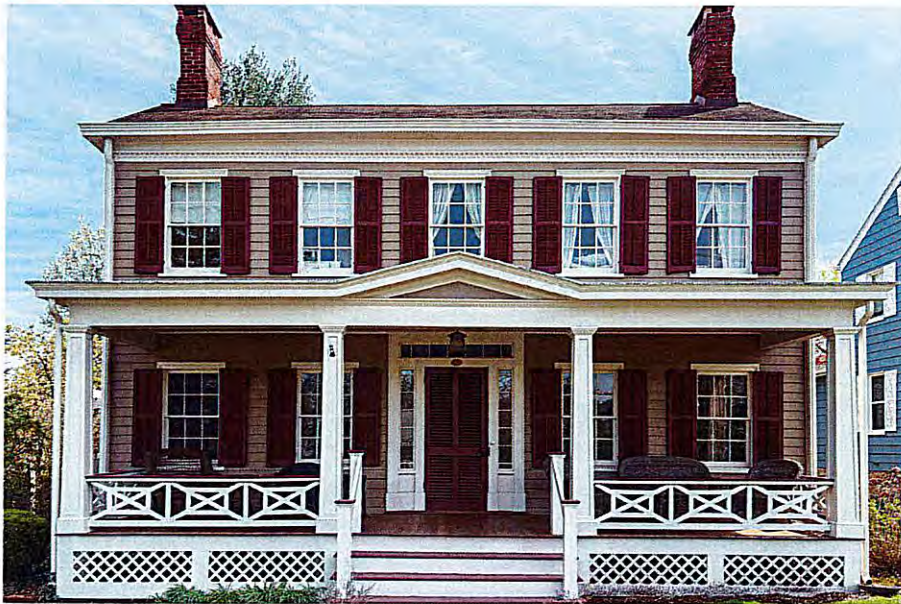
Regularly spaced, double-hung wood sash windows with divided lights and operable shutters are defining features of this symmetrical Greek Revival-style façade with a later Colonial Revival porch
