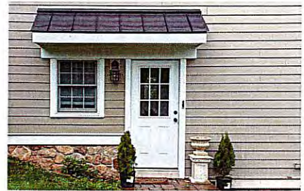
New entry with simple divided-lite door and minimal trim
