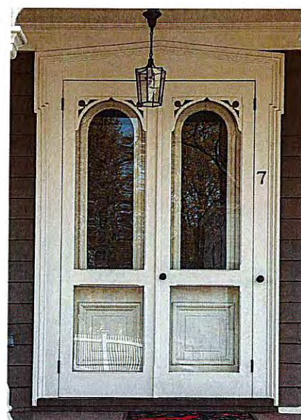
Double-leaf storm doors with arched glass panels reveal wood paneled door behind
