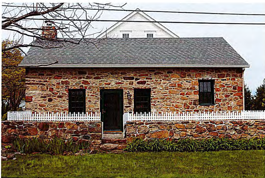
This rubble stone dwelling with minimal ornamentation exemplifies early vernacular construction, where local materials and masonry skill defined both form and function
