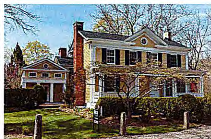
Rear addition is clearly subordinate and set back, preserving the primary façade's prominence
