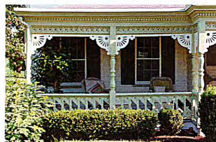
Porch pediment with sunburst panel within decorative sawn brackets accentuated by dentil molding
