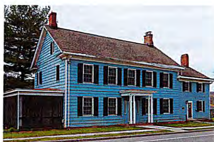
59 Old Turnpike Rd
