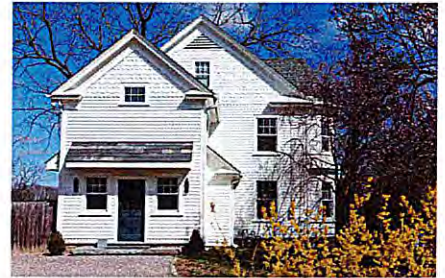
Reconstruction of wing following a fire respects house's original design intent
