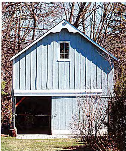
Vertical wood siding and arched loft window maintain traditional proportions in this sensitively rehabilitated garage barn
