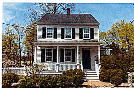
Example of Georgian-influenced local vernacular 10 Church St
