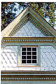
Decorative gable with patterned shingles
