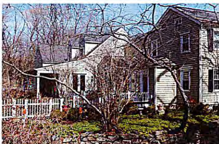
Rear addition does not call attention to itself and is minimally visible from the street
