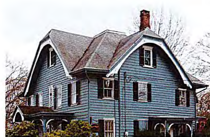
Jerkinhead roofs combine gable and hip roof forms
