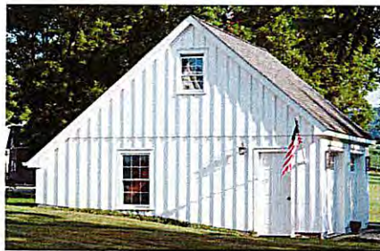
Outbuilding with board-and-batten siding
