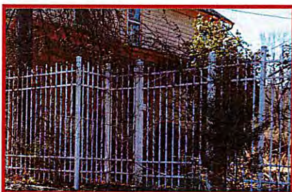
X Inappropriate Ornamental metal fencing with industrial-style detailing is out of character for residential historic districts
