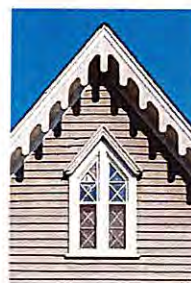
Pointed window & bargeboard trim
