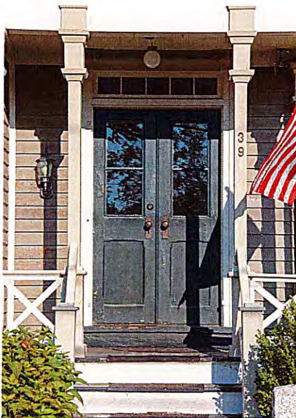
Victorian double-leaf door with transom, framed by simple posts and railings
