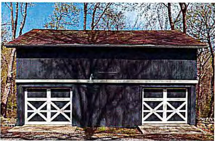
Replace significantly deteriorated primary roofs in-kind or to match the historic original
