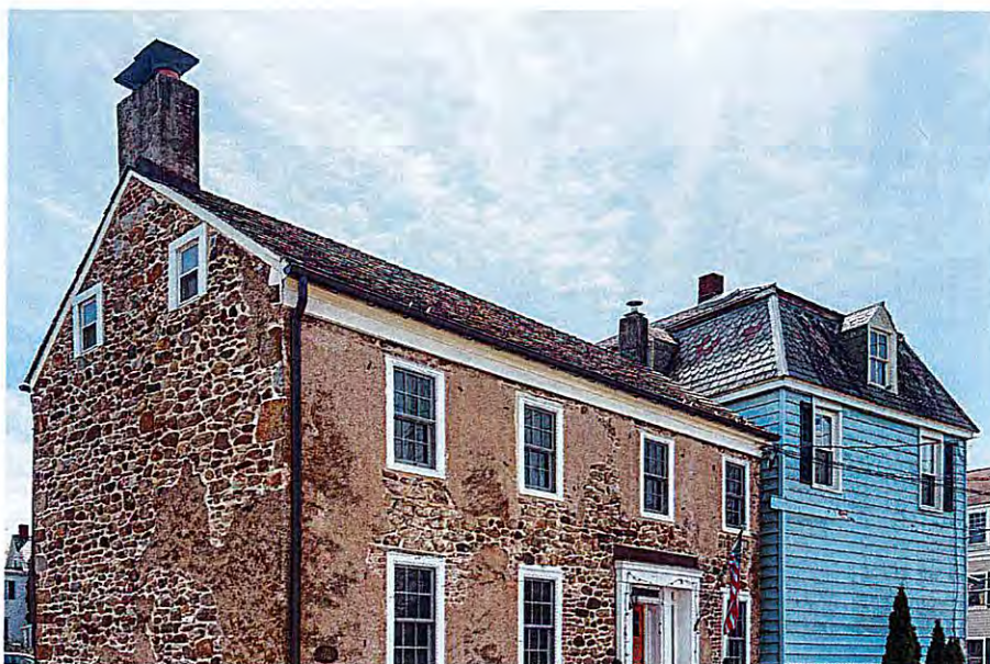
A variety of historic roof forms, materials, and details—such as slate gables and mansards—contribute significantly to the character of Tewksbury's historic districts
