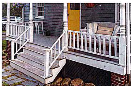
Painted wood decking and simple balustrades contribute to the character of this Victorian porch
