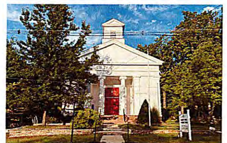
Cokesbury Methodist Church 230 Cokesbury Rd
