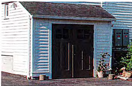
Properly-scaled paneled wood replacement doors reflecting original utilitarian character
