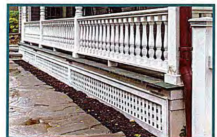
✓ Appropriate Preserve turned balusters and framed wood lattice skirting below
