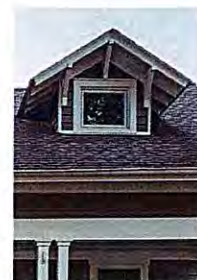
Gable dormer with wide overhang
