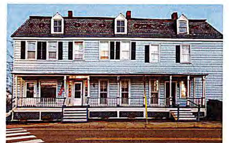
54 Old Turnpike Rd
