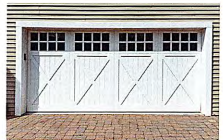
New garage door with paneled appearance and transom references carriage house doors
