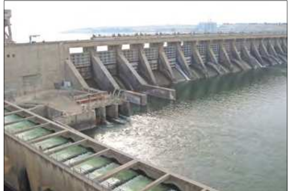
McNary Dam is a 1.4-mile long concrete gravity run-of-the-river dam which spans the Columbia River. The fish ladder is show in the foreground.
