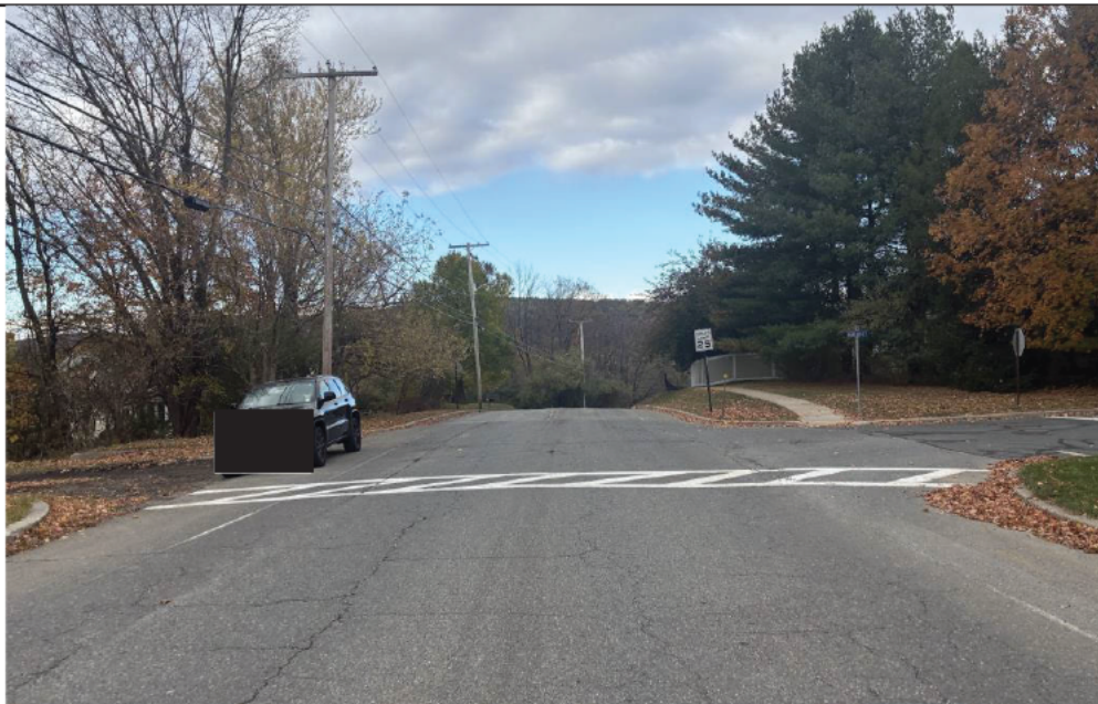
Photo 8: Road to be resurfaced and restriped. Compliant ADA ramps installed with pedestrian activated flashing crossing signs.
