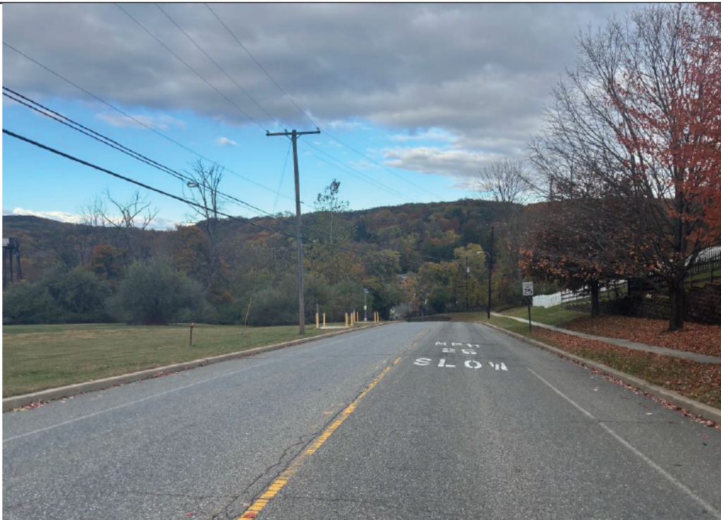
Photo 7: Roadway to be resurfaced and restriped. Sidewalk repaired as needed.
