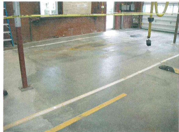
Apparatus bay of concern
