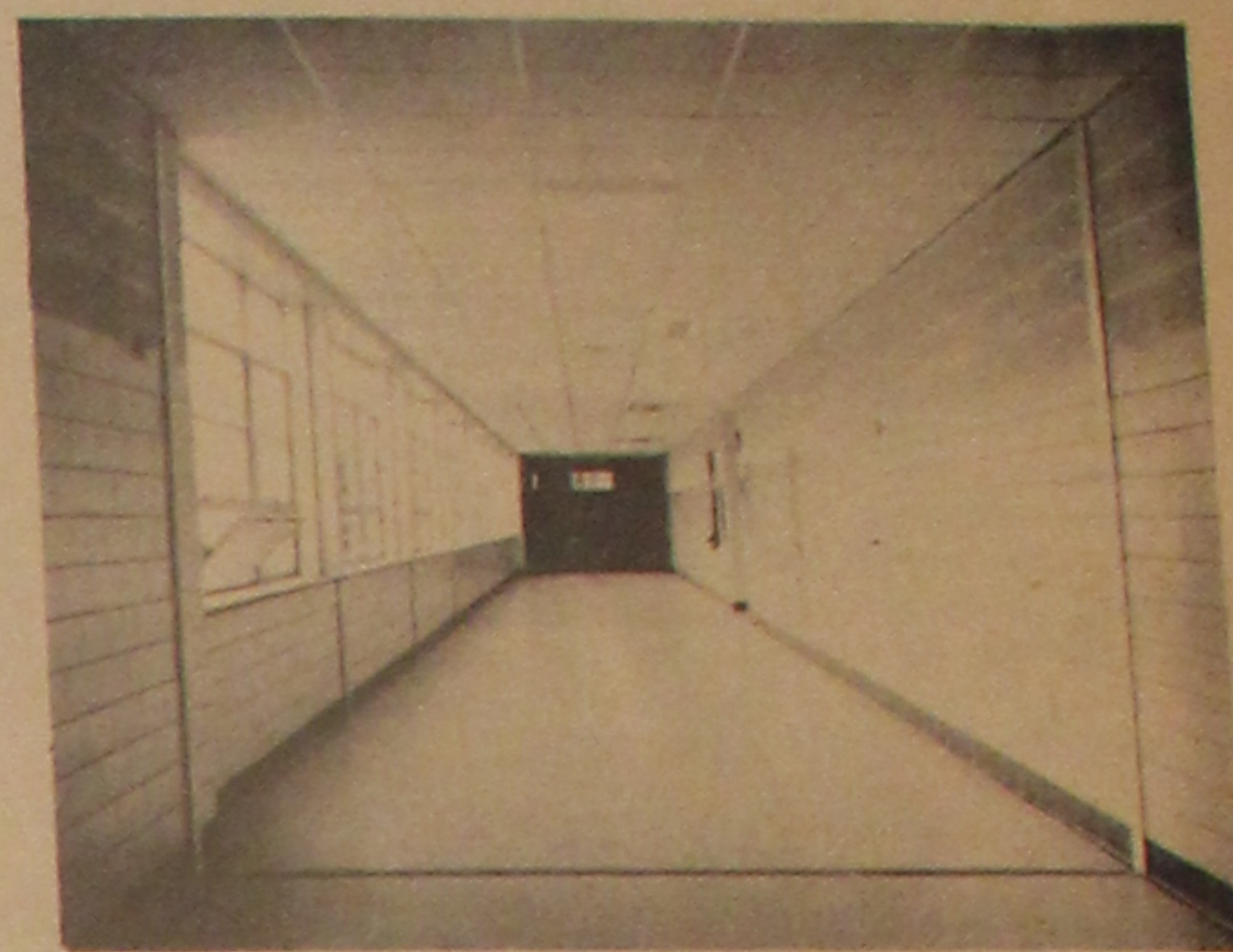
WELL LIGHTED HALLWAYS PROVIDE MAXIMUM OF SAFETY - PREVENT CONGESTION
