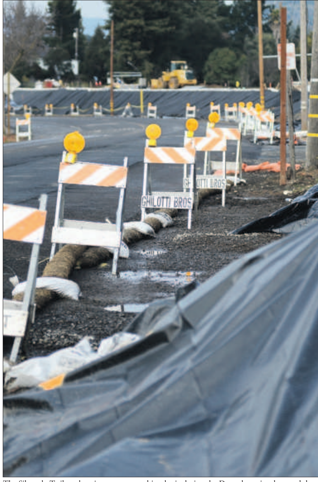
The Silverado Trail road project was wrapped in plastic during the December rains, but work has resumed with drier weather. Lisa James/Register
