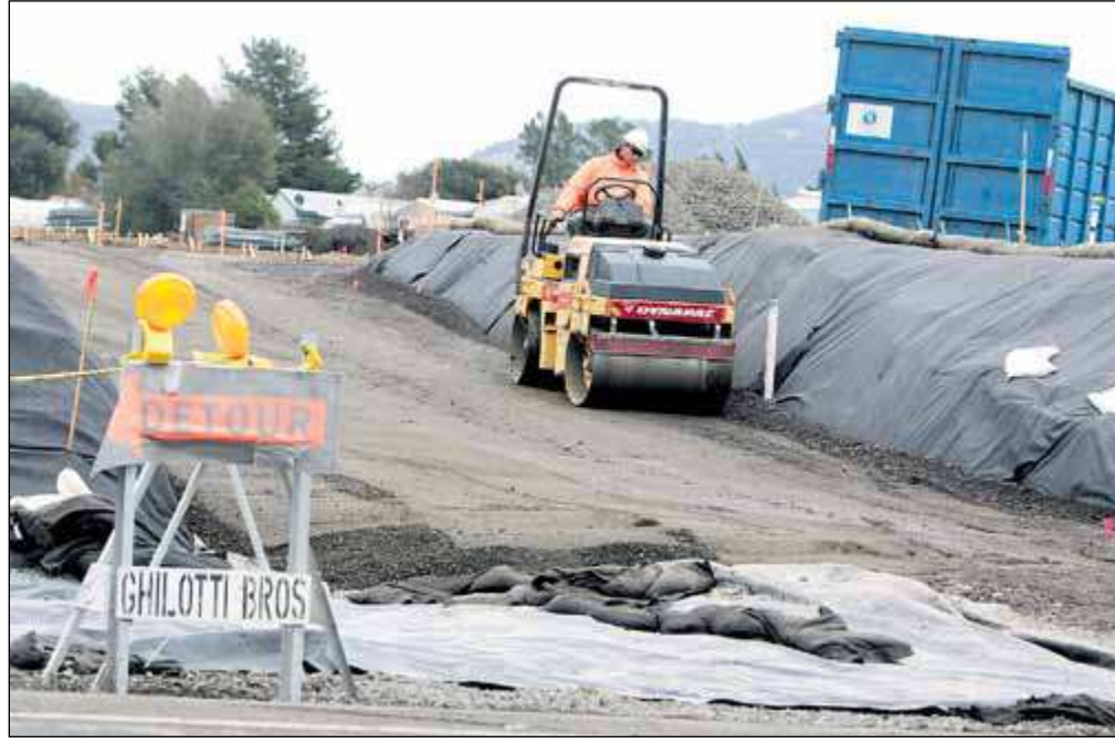
Construction has begun at Alexander Crossing, the 134-unit apartment complex being built along Silverado Trail near Soscol Avenue. J.L. Sousa/Register
