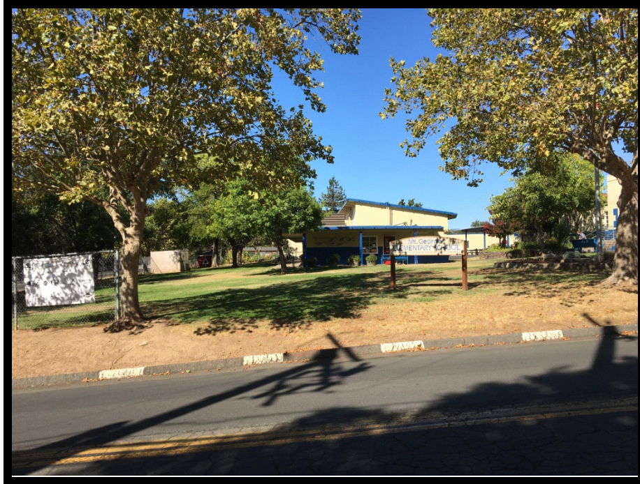
Classroom building from 2nd Avenue
