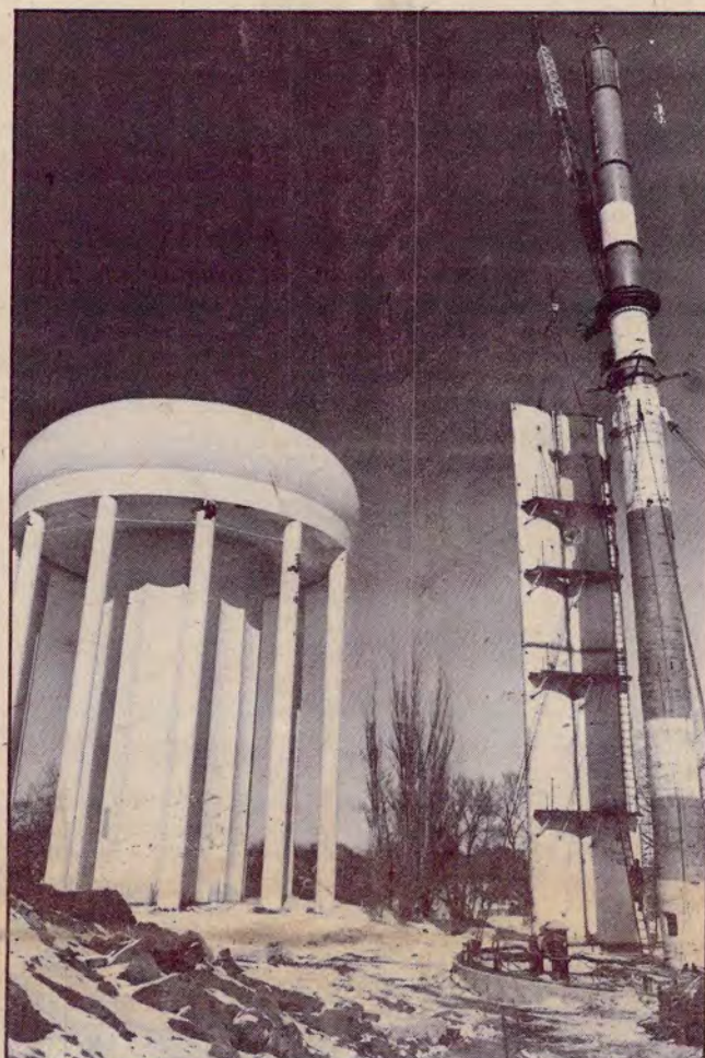
ures a section of the tank's fluted support column—a small fraction of the 25,000 pounds of steel that will be used in the project, scheduled for completion July 1.
