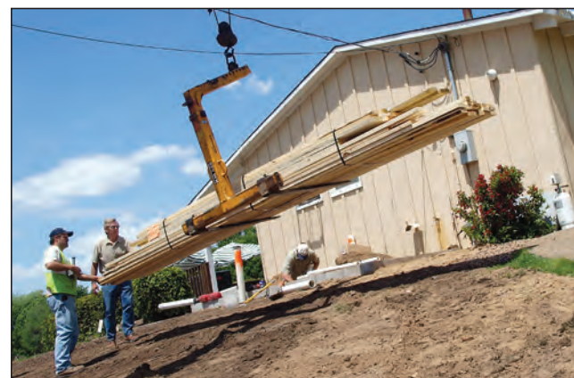
Workers unload lumber for making the clubhouse more handicapped-accessible. PHOTOS BY BRAD STAUFFER
