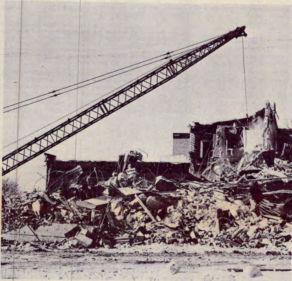
The old St. Therese's elementary school at Prior Avenue and Mississippi River Boulevard fell to the wrecking ball earlier this month. Brutger Companies is planning to erect a three-story, 54-unit apartment building on the site.
