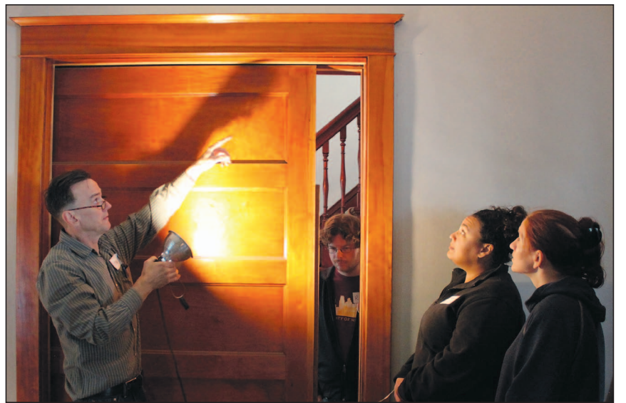
Instructor Ezra Gray teaches students at a home in St. Paul how to repair a pocket door that does not open and close smoothly. PHOTO COURTESY OF RETHOS
