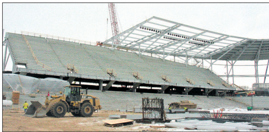
A view of the bleachers going up at the new Allianz Field soccer stadium that is under construction in the Midway. PHOTO BY LOU MICHAELS
