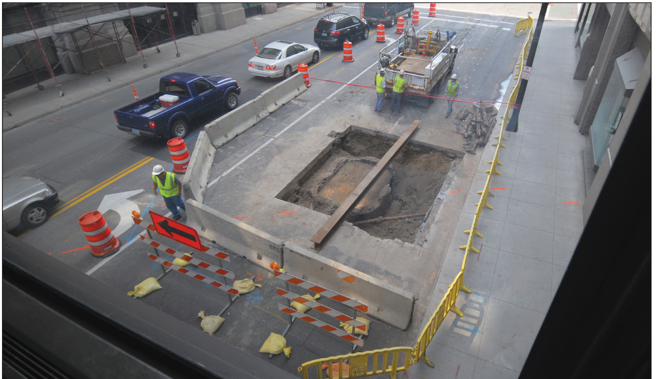
Utility work is under way at 4th and Robert streets in downtown St. Paul in preparation for construction of the proposed Central Corridor light-rail transit line. PHOTO BY ANNE BRANDRUD
