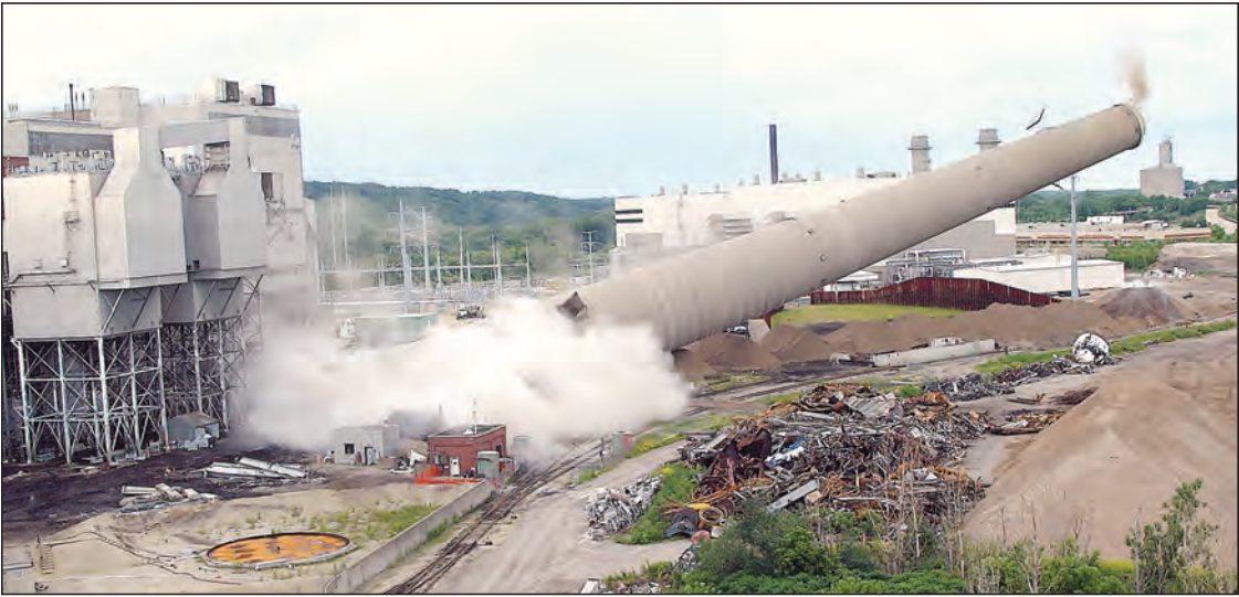
The 570-foot-tall smokestack of Xcel Energy's old High Bridge plant nears the ground after being imploded on June 28. The new power plant is pictured in the background. PHOTOS BY BRAD STAUFFER
