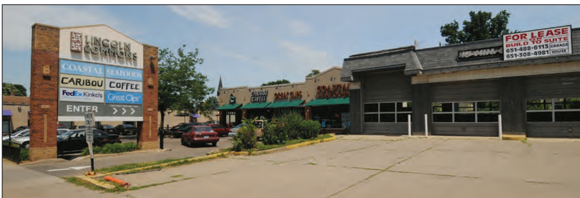
A new Sherwin-Williams paint and decorating store is planned for the northeast corner of Snelling and Lincoln avenues, on the former site of an auto lube business. PHOTO BY ANNE BRANDRUD
