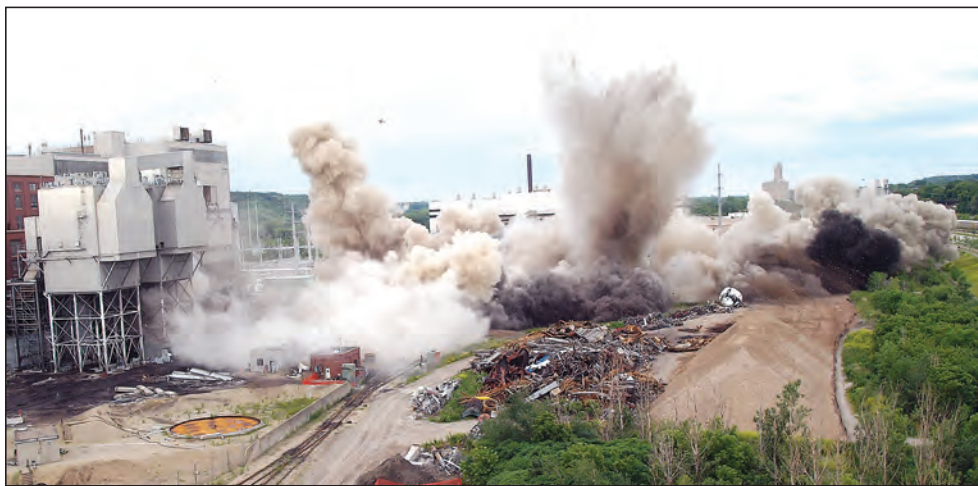
A huge cloud of dust and debris leaps from the site of smokestack implosion.
