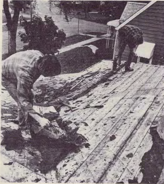
Roofers tear off the old shingles and waterproof felt from the top of a residence on Middleton Avenue.
