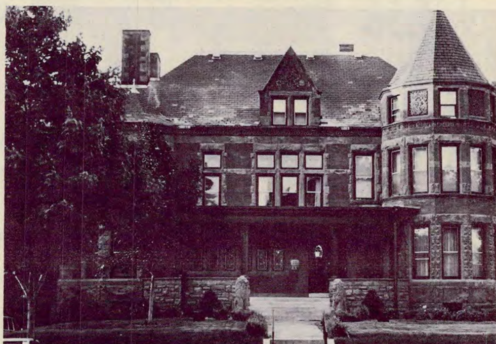
The stone mansion at 332 Summit Ave., built in 1889, was designed by state Capitol-architect Cass Gilbert in the Richardson Romanesque style.
