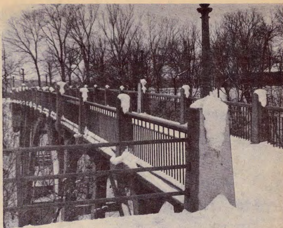
Posts on the footbridge over Montreal Avenue don their stocking caps in preparation for the long winter ahead.
