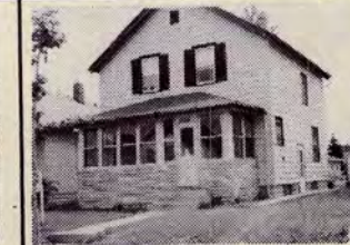
2 story, 3 bedroom, much updating done. Formal dining rm, maint free exterior newer furnace. Viki Felden - Montague 699-6666
