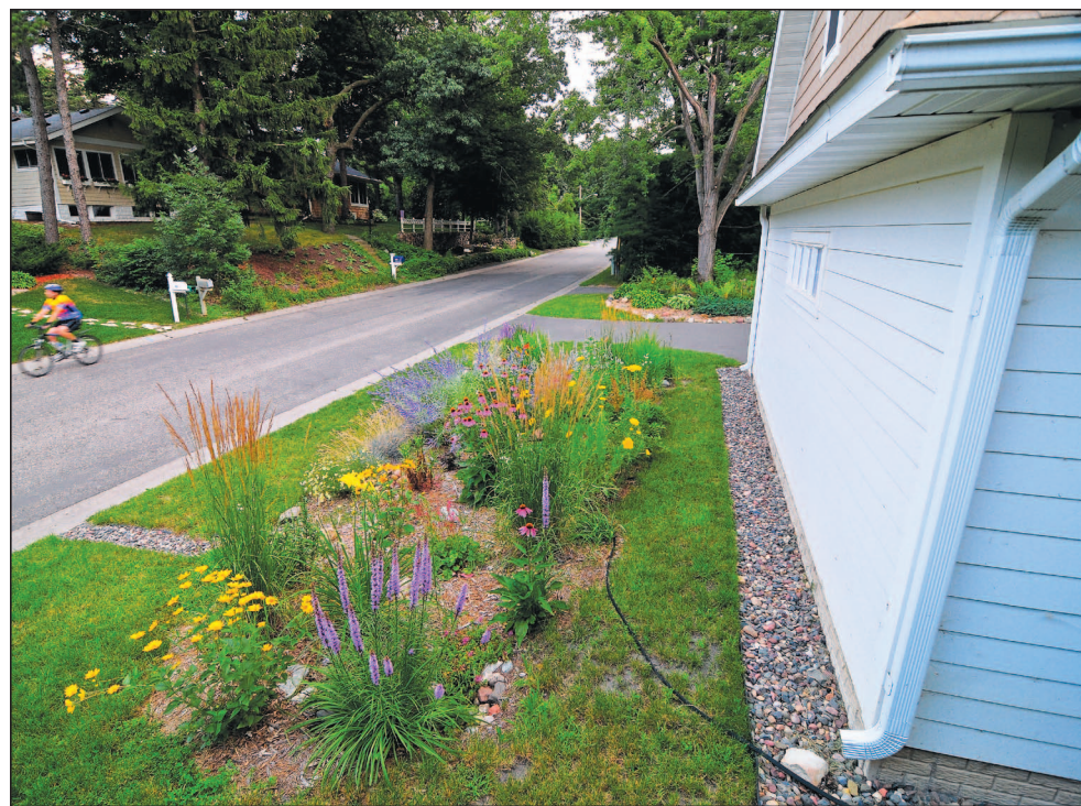
A rain garden of native plants captures the stormwater runoff on the side of this home.
