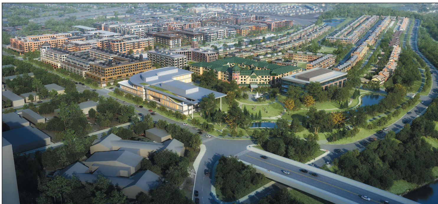
With an estimated value of $40 million now, the 122-acre Ford site in Highland Park is expected to be worth $1 billion when fully built out over the next two decades with new housing, retail, office and institutional uses as pictured above looking toward the southeast.
