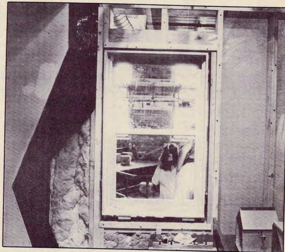
The Children's Museum's hands-on exhibit, "About the House," cuts through the wall of a typical house to expose layers of sheetrock, plastic, insulation and studwork.
