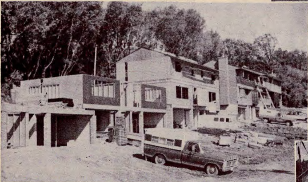
These three-story townhouses (above) are going up near the corner of Morgan and Davern.
