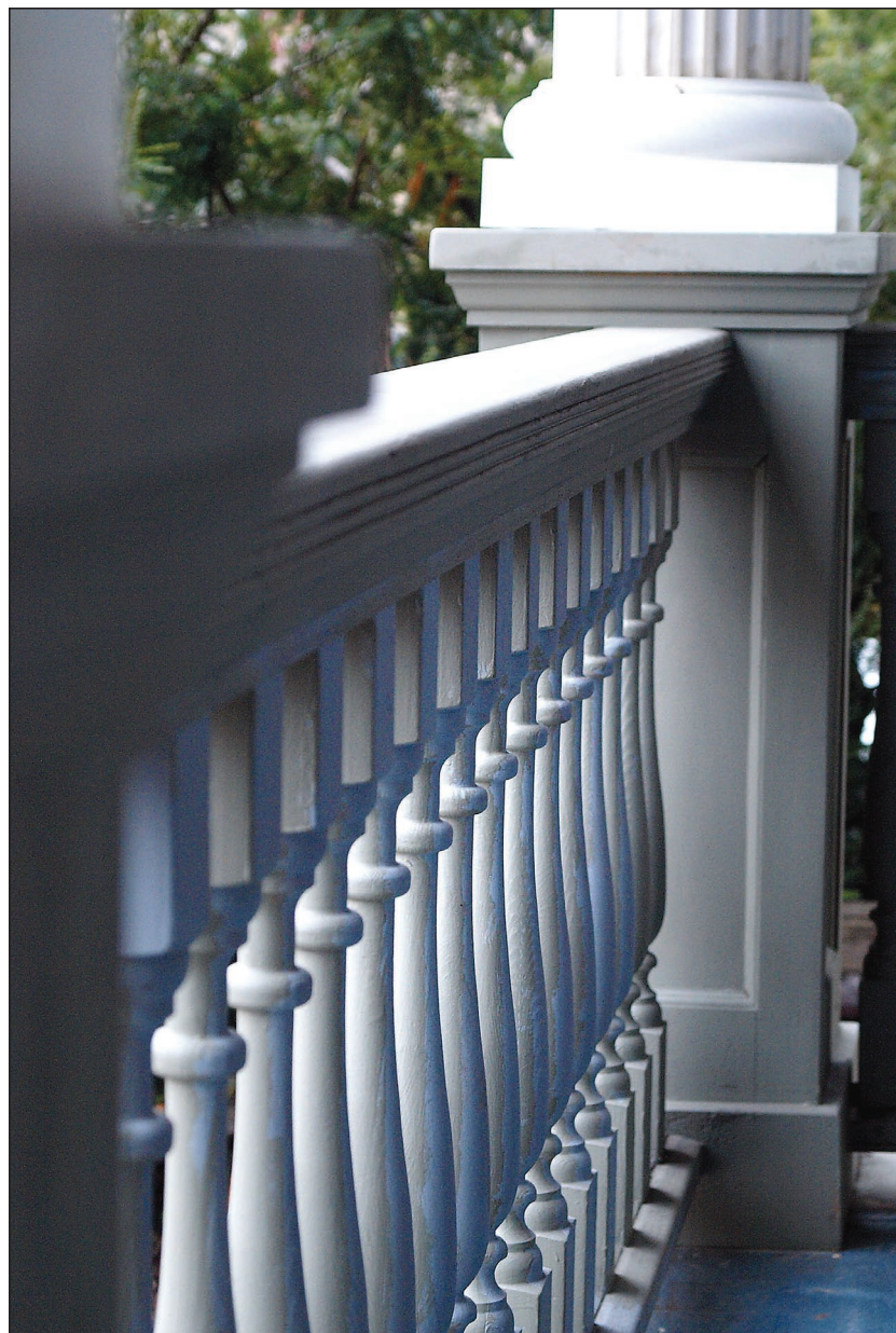
The spindle railing on the Theverapperuma's newly open front porch.
