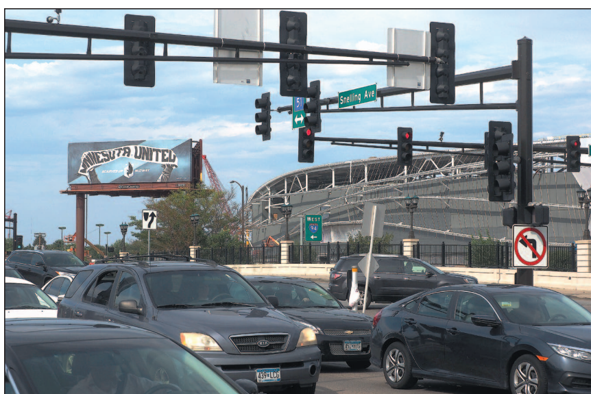
Traffic buzzes by the Major League Soccer stadium under construction on the northeast corner of Snelling and St. Anthony avenues. PHOTO BY BRAD STAUFFER
