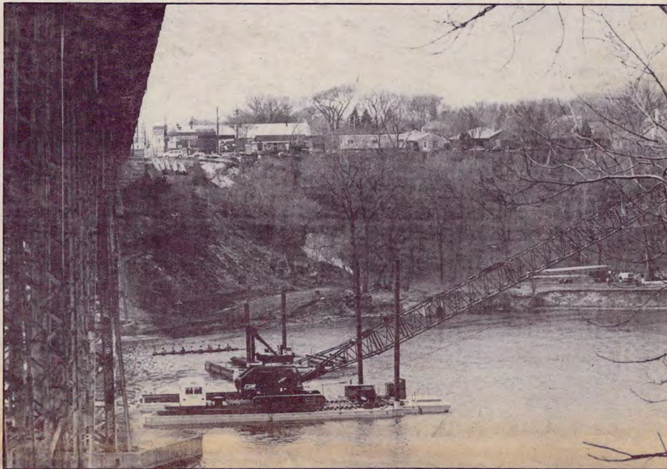
The long-awaited project to replace the Lake Street-Marshall Avenue Bridge finally began last week with the clear-
