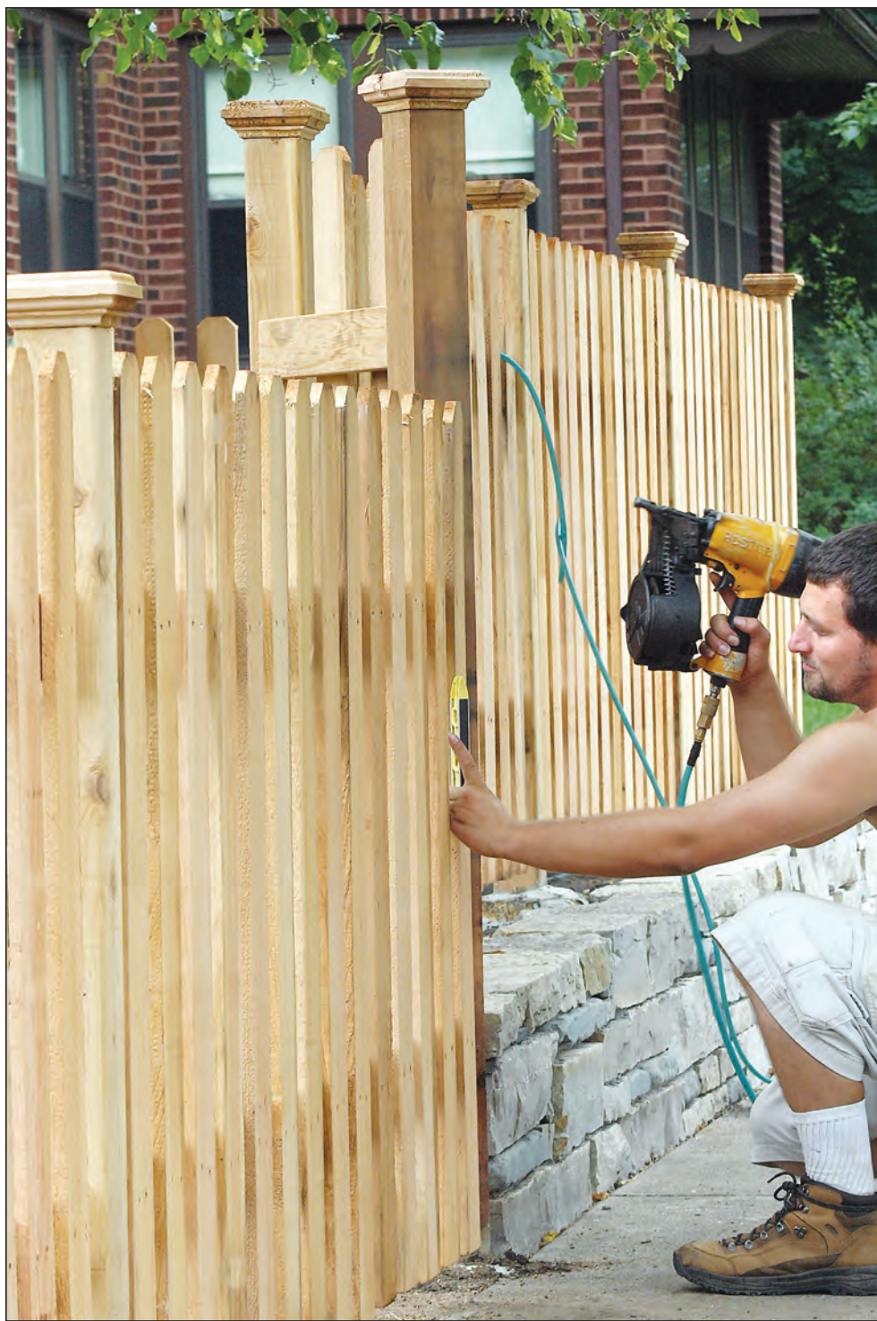
Cedar boards are nailed in place by Premier Fence installer Jesse Stoker at a home in the Summit Hill neighborhood. PHOTO BY BRAD STAUFFER
