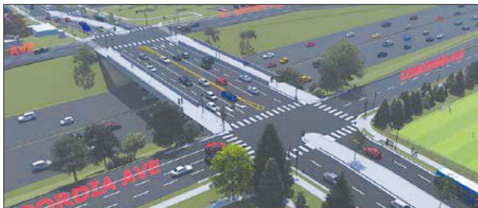
The Dale Street bridge over I-94 (seen from the southwest) will be reconstructed in 2020 with two 16-foot-wide pedestrian plazas and more room for bicycles and cars.
