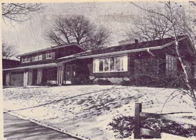
Breck School's Idea House, at 4848 Northrop Drive in Minneapolis.
