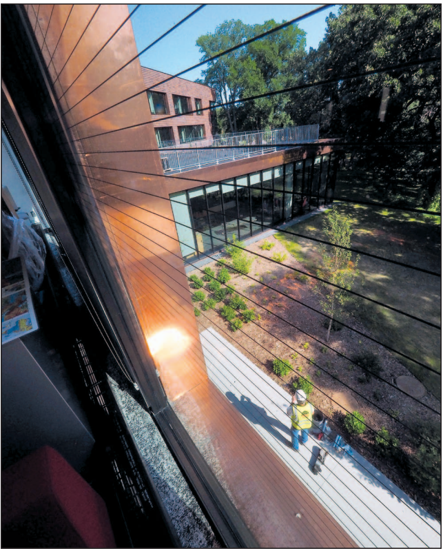
A second-floor view of the library and fenced rooftop where a garden will be installed at Minnehaha Academy’s rebuilt Upper School. PHOTO BY BRAD STAUFFER
