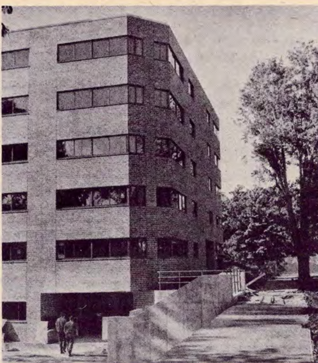
With only surrounding cosmetic work still to be completed, St. Thomas' new student residence opened to 144 female students on Labor Day.
