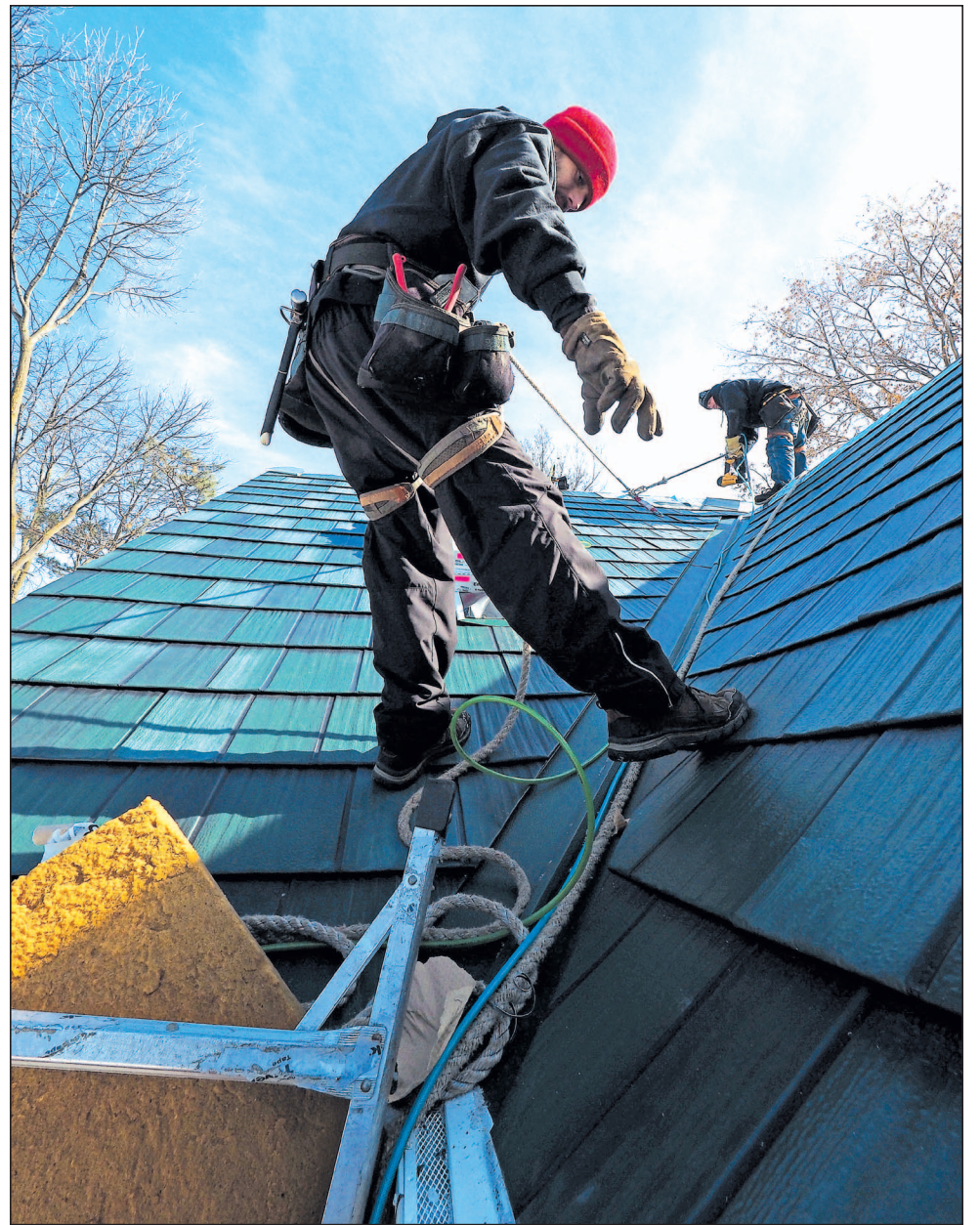
Mike Harrison and Roger Williams of Quarve Contracting install a new architectural shake-style metal roof on a Macalester-Groveland home. Pictured at left is the roof nearly completed. PHOTOS BY BRAD STAUFFER
