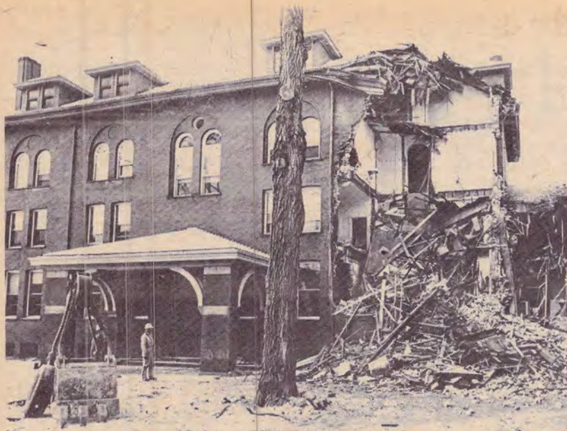
A wrecking crew made short work of a landmark structure on the St. Paul Seminary campus last month. The old administration building, designed by St. Paul ar-
