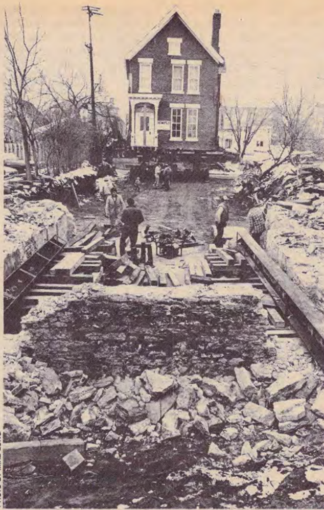
This house, which until the week before Christmas was located at 727 Grand Ave., was moved just across the alley to a lot owned by Nancy White, who lives next door at 726 Summit Ave. Nancy and her husband Doni bought the house from Inco Properties, which removed the house to make way for the planned expansion of the Pier 1 store.
