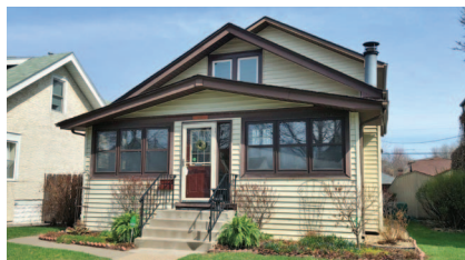
1559 Sargent Ave – Just Listed! Impeccable 4 bedroom 1.5 story! Featuring gleaming wood floors, porch, updated kitchen, finished lower level family room with fireplace & dbl garage! $315,000
