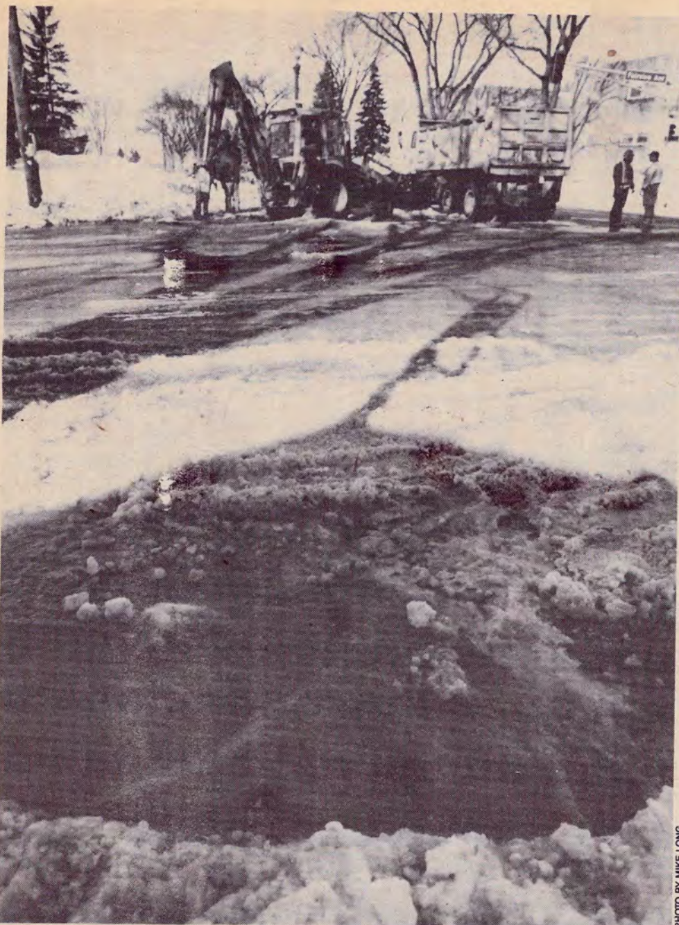
The early-March snowstorm not only dumped a hefty load of snow on the Twin Cities. In the balmy days that followed, rapid melting created small lakes in areas where the storm sewers were clogged with ice and slush. The flooding got so bad at Ford Parkway and Fairview Avenue that city crews were called out to clear the storm sewers of obstructions. The water was soon flowing again.
