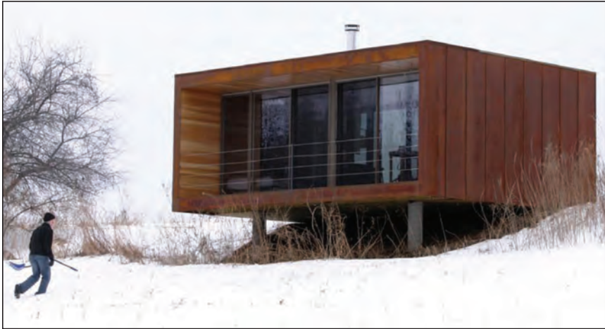
The Arado weeHouse that started it all in 2003. PHOTO FROM ALCHEMY ARCHITECTS
