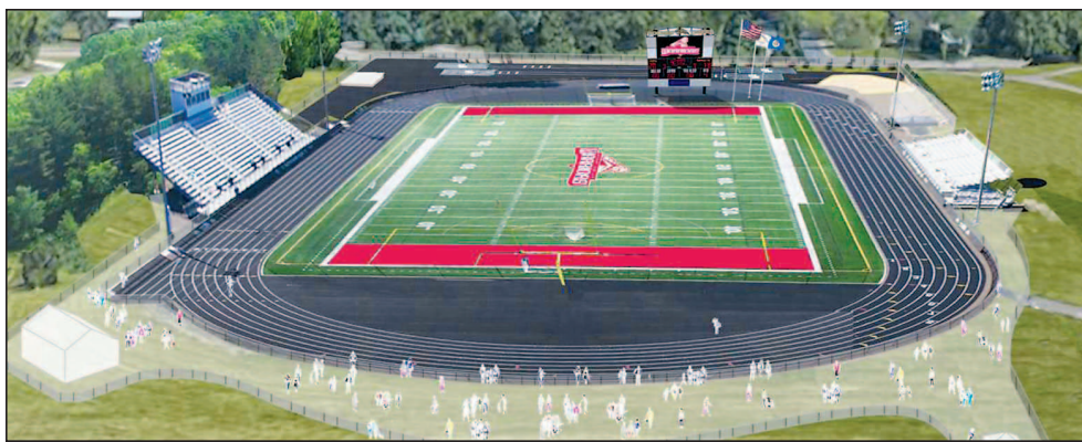
Groundbreaking is expected to take place soon on Sibley's new multipurpose field.
