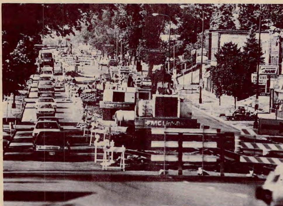
As if driving in the recent heat weren't enough fun, sewer reconstruction work has reduced Snelling Avenue to two lanes between Randolph and Fairmount avenues. The project is expected to last through the end of the month.
