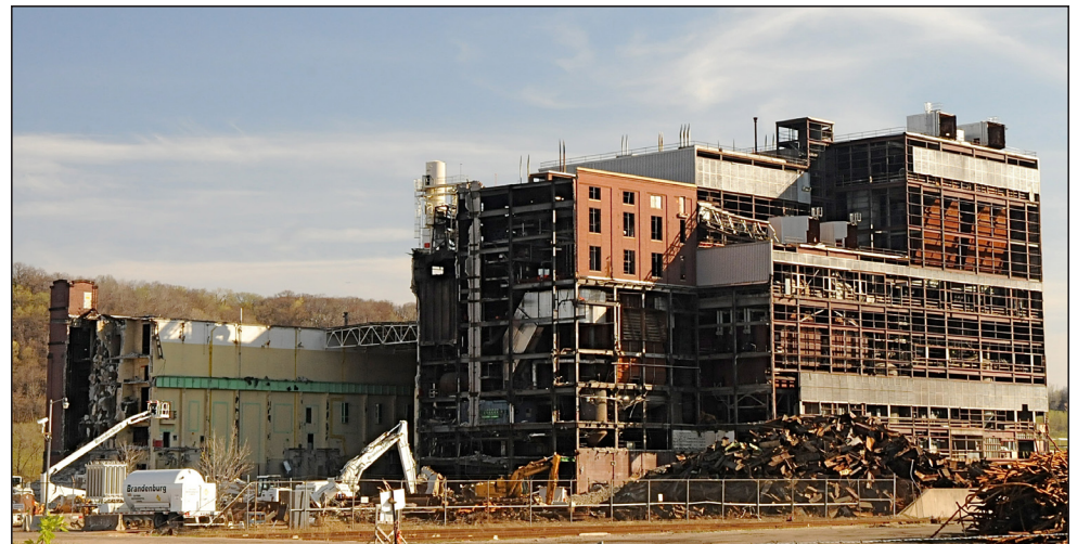
Slowly, but surely, Xcel Energy's old coal-fired High Bridge plant continues to be dismantled. Its 570-foot-tall smokestack has been gone since last June. PHOTO BY ANNE BRANDRUD
