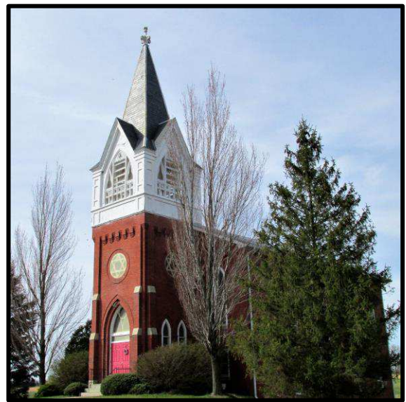
Figure 13: Villages contain many important architectural examples
