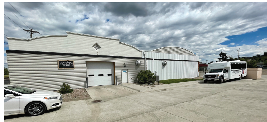
NTI facility with the new concrete driveway which was installed last year with Cares Act funding Photo Credit: NTI
