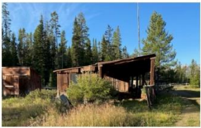
TRAILER STRUCTURE TO BE REMOVED
