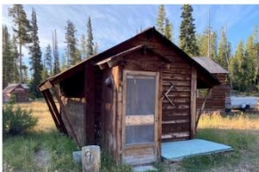
CABIN # 9 TO KEEP, MAINTAIN AND REPURPOSE
