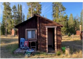
CABIN # 4 TO BE REMOVED
