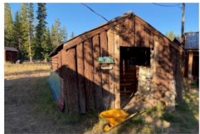
CABIN # 6 TO BE REMOVED
