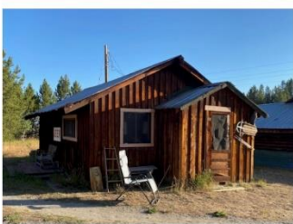
CABIN # 3 TO KEEP, MAINTAIN AND REPURPOSE
