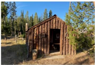
CABIN # 5 TO BE REMOVED
