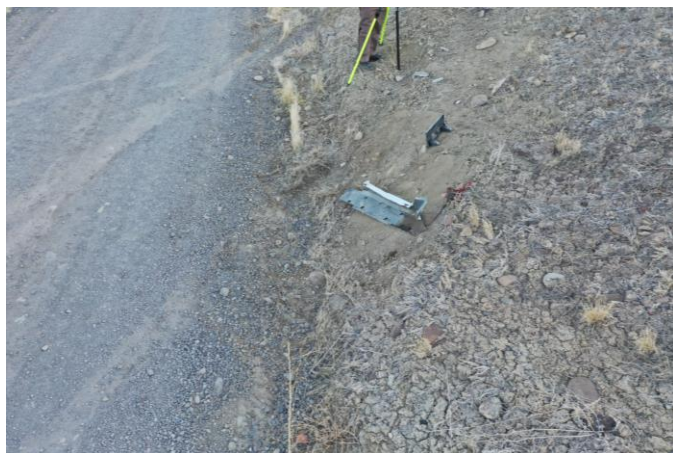
Exhibit 1 – Debris on Hidden Springs Road
