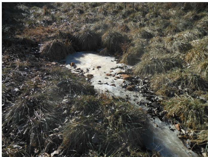
Photograph: # 17. Taken By: Joe Trunko Date Taken: January 13, 2022 Program: WMP-RCRA D Entity: Generally Hauling Sanitary Landfill Permit: 107104 Location: North slope of landfill Description: Leachate outbreak on lower west side of north slope.
