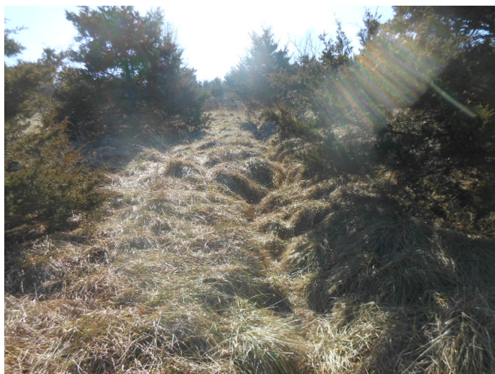
Photograph: # 15. Taken By: Joe Trunko Date Taken: January 13, 2022 Program: WMP-RCRA D Entity: Generally Hauling Sanitary Landfill Permit: 107104 Location: East side of North slopr Description: Erosion ditch located in the central section of the east side of the north slope; looking south upslope.
