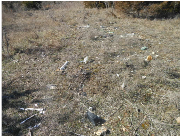
Photograph: # 14. Taken By: Joe Trunko Date Taken: January 13, 2022 Program: WMP-RCRA D Entity: Generally Hauling Sanitary Landfill Permit: 107104 Location: Central area of landfill Description: Exposed waste sticking out from cover.
