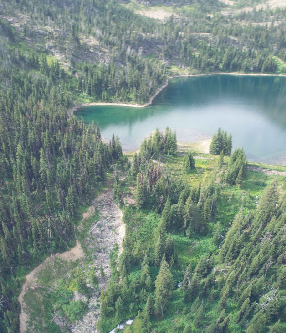
Figure 1. Eroded spillway at McKinley Lake
