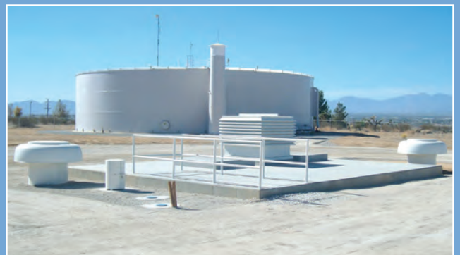
Construction of the Mockingbird Pump Station (top photo) and the completed underground station (bottom photo).
