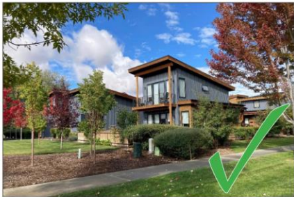
Cottage style dwelling units
