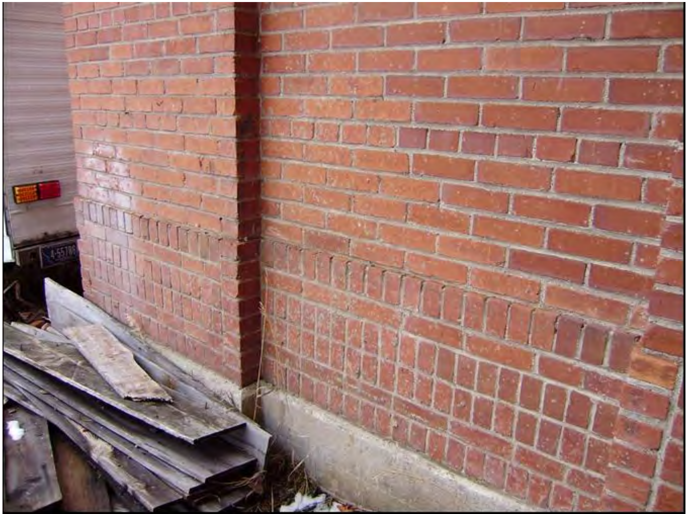
Photo 0016. Detail of brick water table. View to northeast.
