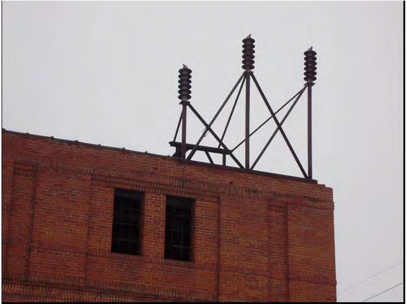
Photo 0018. Detail of lightning arrestors. View to southeast.
