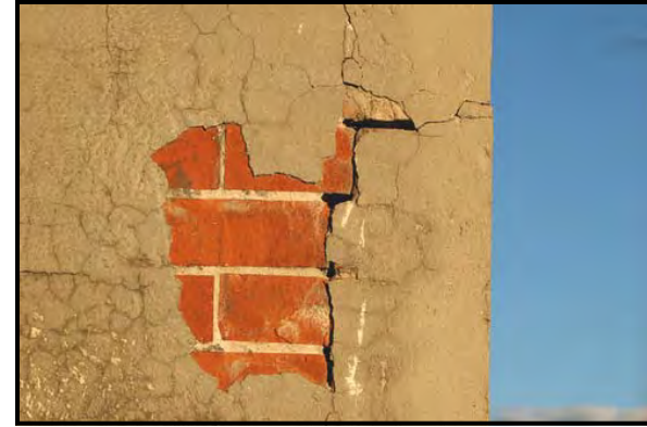
Poor examples of a material choice to repair brickwork
