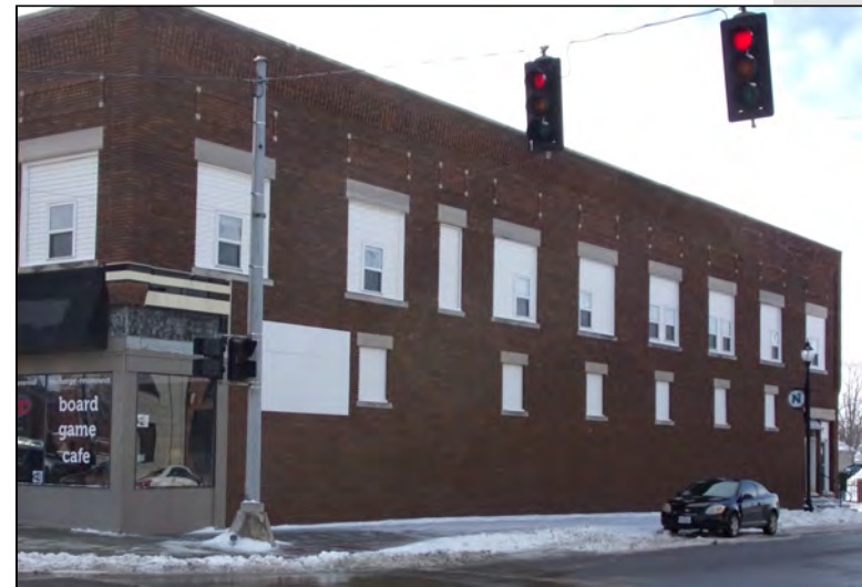
Siding infill and mismatched window openings
